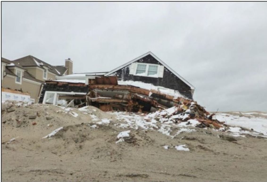
Image #2: The above example photo illustrates pancaking.
